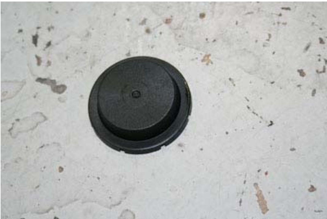
Pulley cover removed
